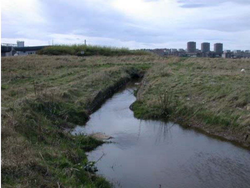
Seawards side exit of East Tullos Burn
